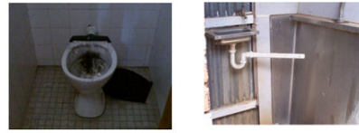
Plumbing (Replacement of fittings and repair of leaks)
